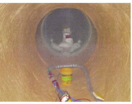
Fig. 6: Robotic sprayed-in-place pipelining
