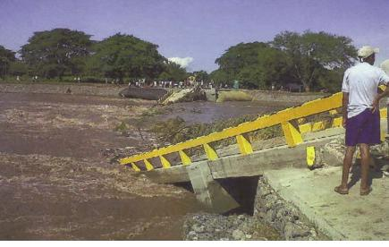
Fig. 4: Flooded river and collapsed bridge in Honduras
